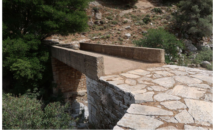
View of Kamilaris Bridge
