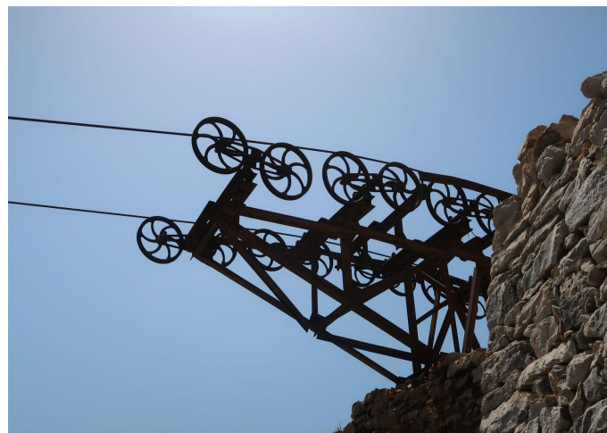
Major junction on the emery cable way
