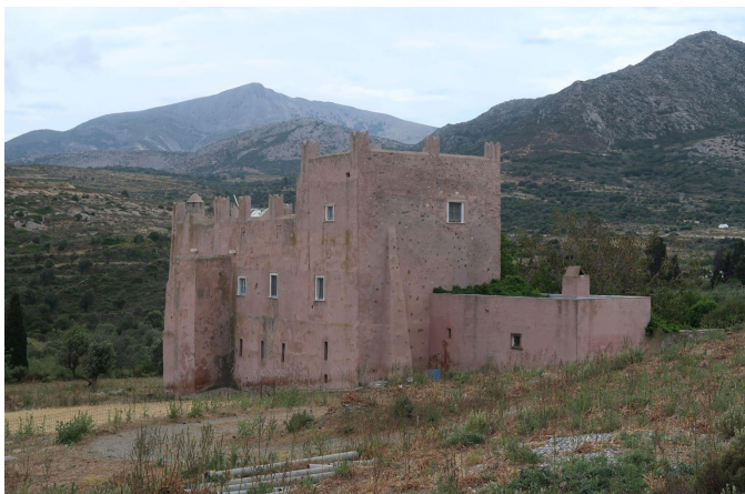
Barozzi Tower House (17th c.)
