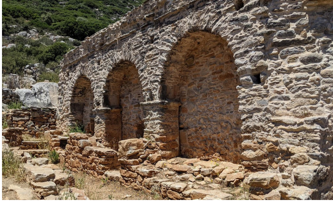
South facing facade of Byzantine Church of Taxiarches Rachi (7th-8th c.)
