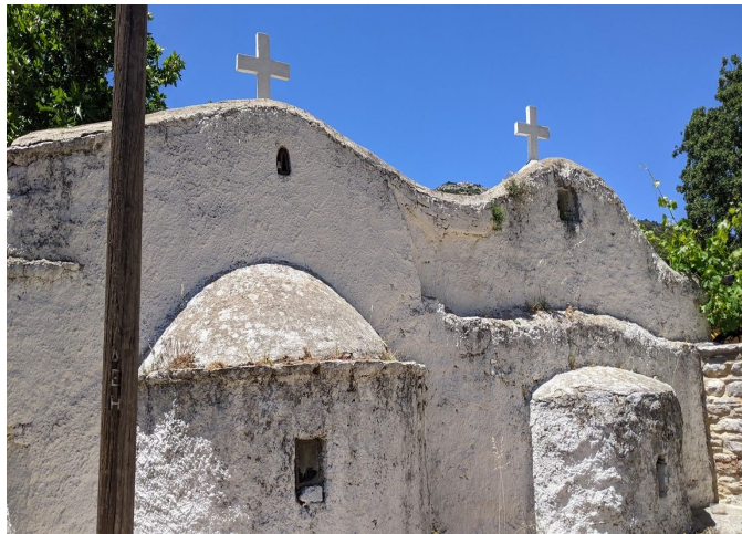
Rear facade of Byzantine Church of Agios Nikolaos-Agios Demetriou (13th c., Monitsia)
