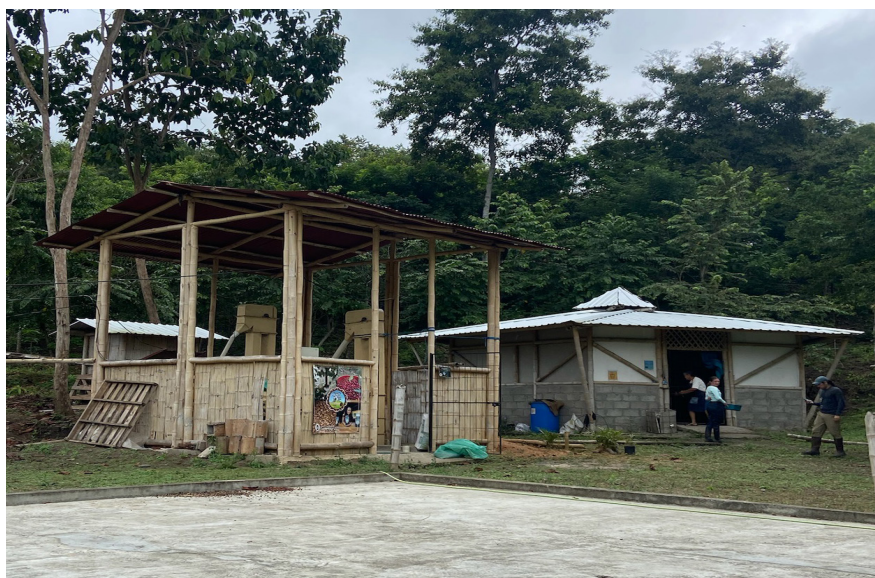
Figure 5.2. Two of the main structures at the ASOPRO Facility
