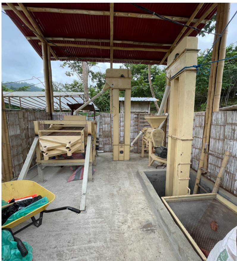
Figure 5.7. Coffee processing equipment at the ASOPRO Facility
