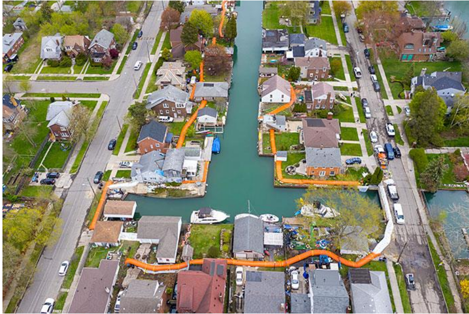
Figure 11: An aerial view of the orange tiger dams in Jefferson Chalmers 47 .
