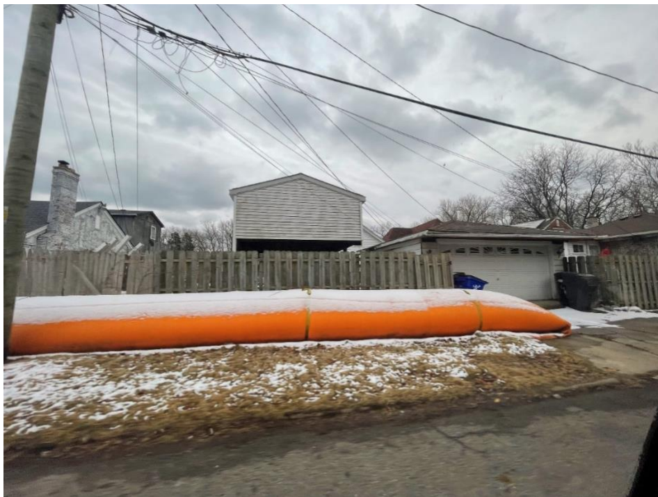
Figure 12 A tiger dam is pictured protecting houses from canal flooding due to high lake and river levels. Photo courtesy of Rachel Woodcock.
