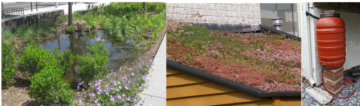
Figure 2 From left to right: illustrations of a rain garden [2], a living roof [3], and a rain barrel [4].
