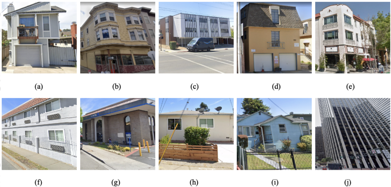
FIGURE 6 Examples of Soft-story and non-soft-story buildings; a-e are soft-story; f-j are non-soft-story
