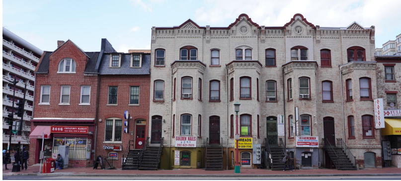
Figure 2: Photo looking north at the H Street NW between 6th and 5th Street NW, Chinatown, Washington, D.C.
