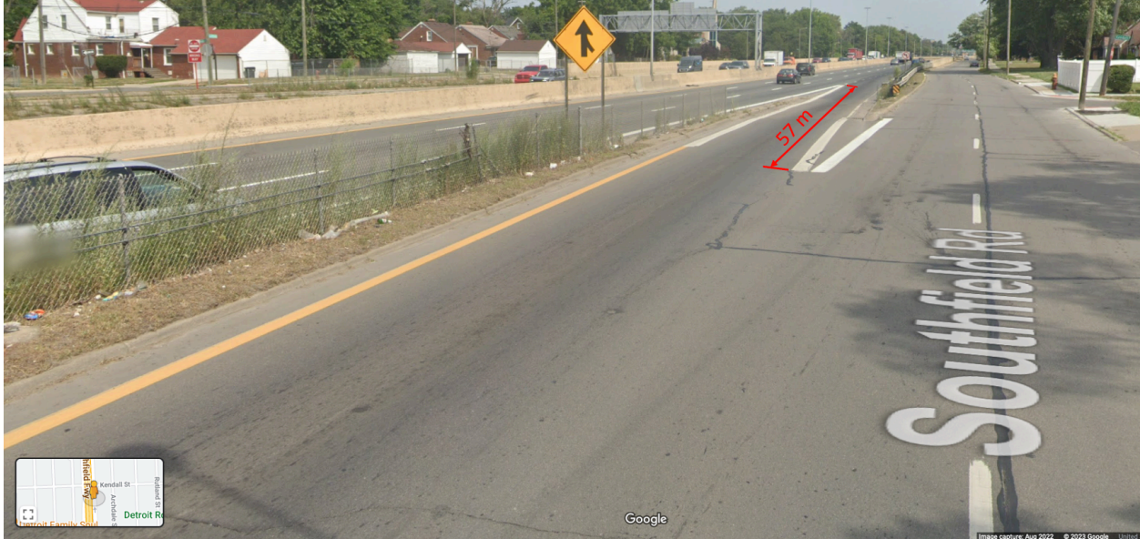
Figure 5: A perspective view that a driver sees entering the on-ramp in Figure 4. The picture point-of-view is from the start of the 100 m on-ramp. The 57 m distance dimension in the picture is from the start of the painted merge line adjacent to the service drive to the end of the painted merge line adjacent to the highway. Image copied from Google Maps, March 6, 2023.
