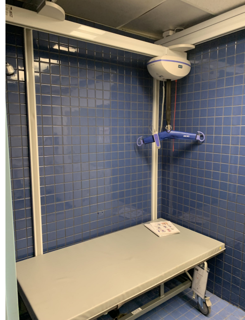
Figure 3. One example of a Motorized X-Y gantry system used in hospitals
