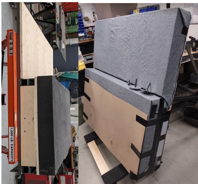
Figure 31. Construction of preliminary side impact load wall.
