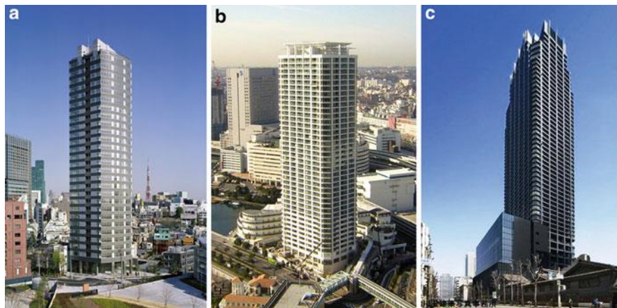
Figure 2.12: Buildings with ECC coupling beams: (a) 27 story Glorio-Tower, Tokyo, (b) 41 story Nabule Yokohama Tower, Tokyo, and (c) 60 story Kitahama Tower, Osaka. [7]
