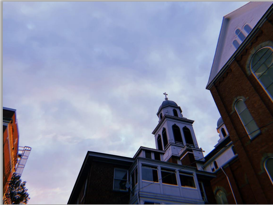
Figure 39. View from outside the National Pinoy Archives, which shows the Immaculate Conception Catholic Church, right next door. The building that houses FANHS National Pinoy Archives was formerly the Catholic school belonging to Immaculate Conception Church, but has since been transformed into a space for the FANHS National Pinoy Archives. Source: Field photograph by author on August 10, 2023. Seattle, Washington.
