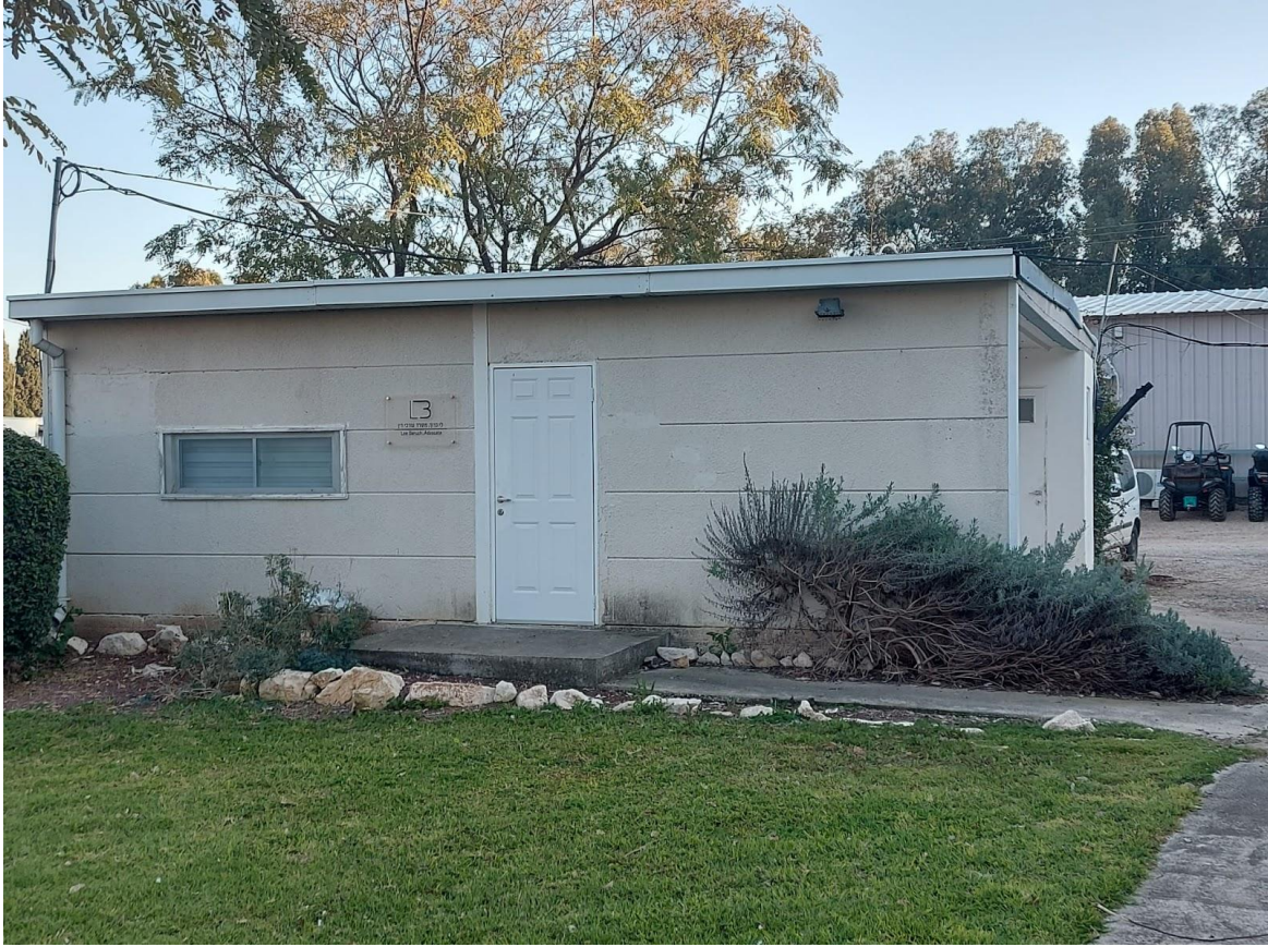
Figure 12 A private lawyer's office in the old collective electric workshop. Photograph: Omri Senderowicz, 2020.
