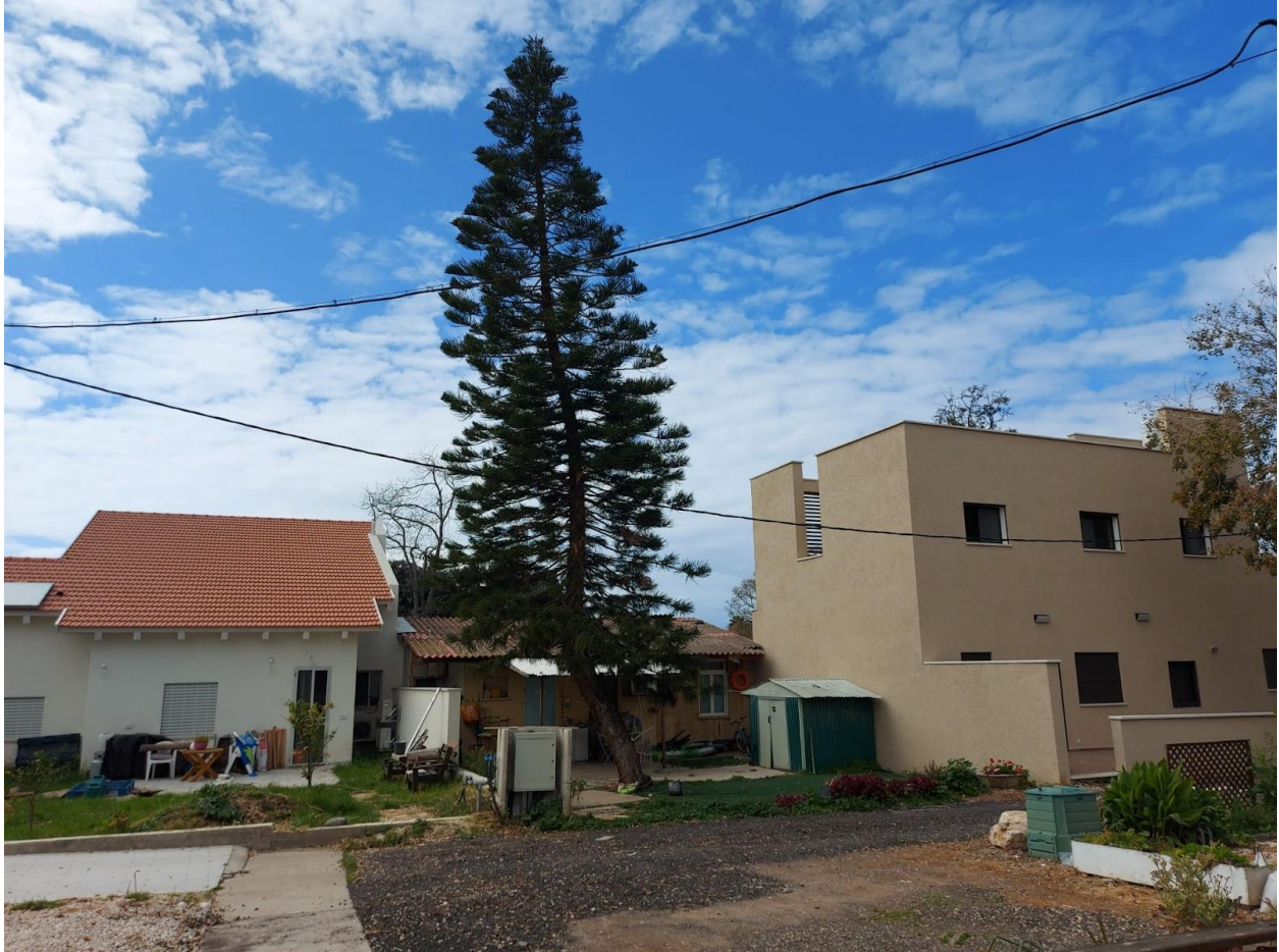
Figure 18 A fragmented “train” house. Ya’ara, a veteran female member, calls this block in the kibbutz: “Yesterday, Today, Tomorrow.” Yesterday is the original “train” apartment in the middle. Today is the one on the left: a new, bigger, yet still “kibbutz-like” home. Tomorrow is the one on the right: “too big and extravagant” in the eyes of the veteran kibbutzniks. Photograph: Omri Senderowicz, 2020.
