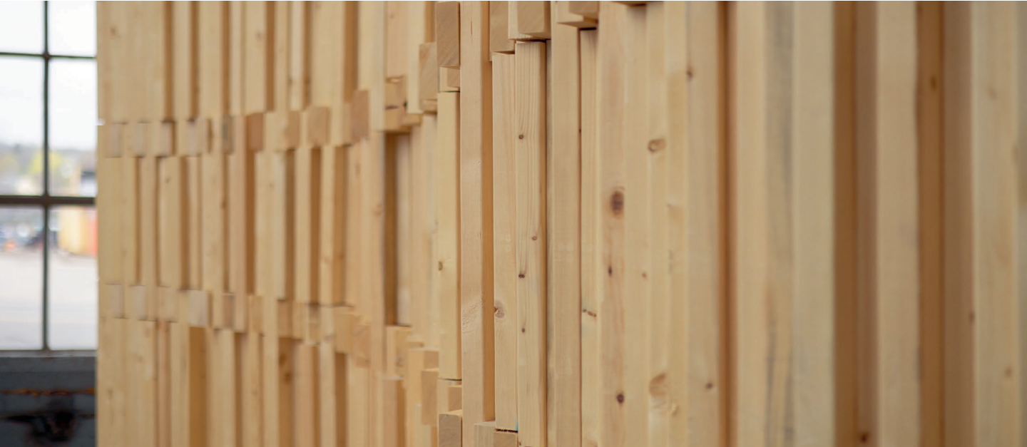
1 Bespoke nail-laminated timber construction.
