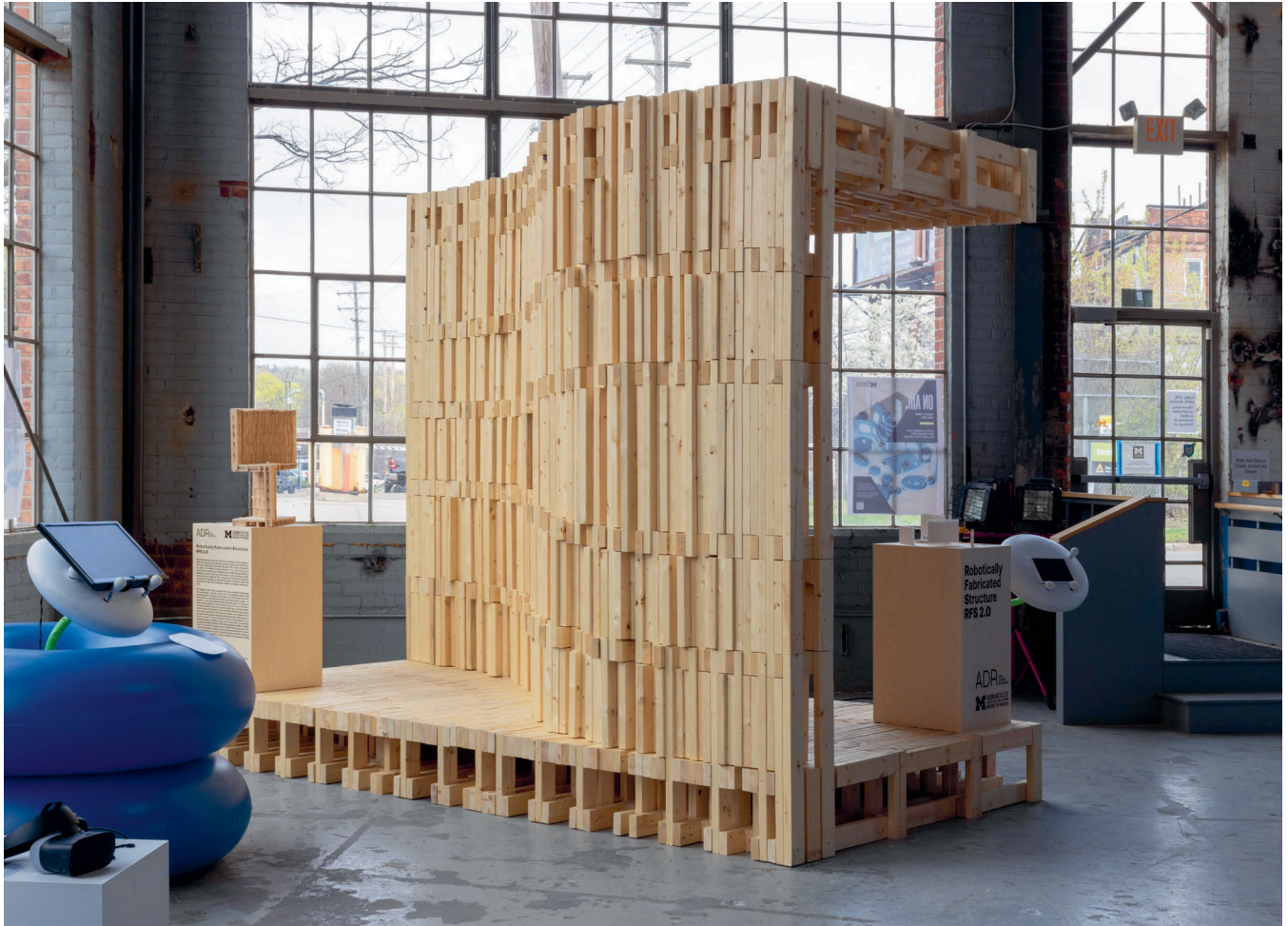
5 Fully assembled NLT structure, showing exterior wall and cantilever roof.
