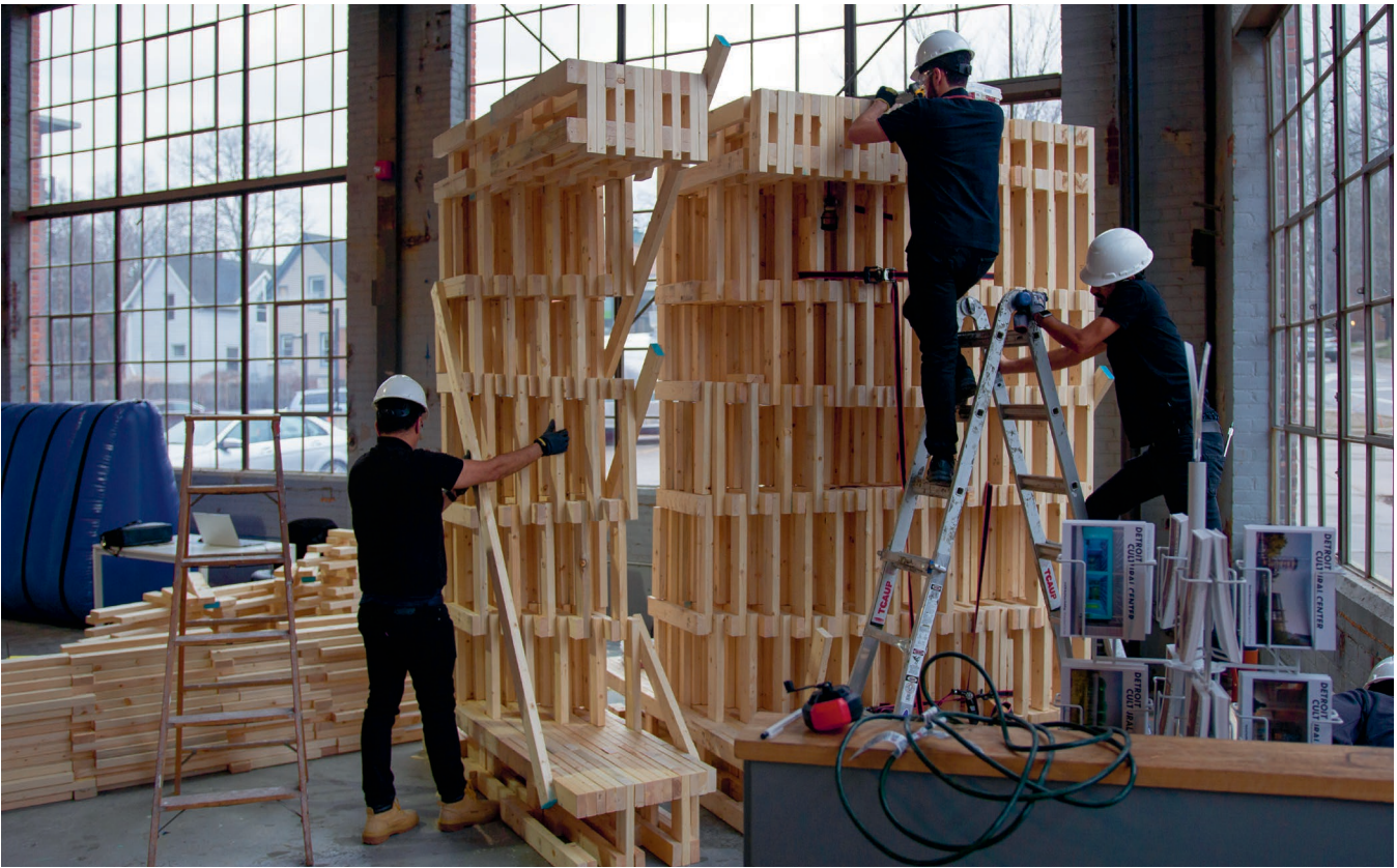
4 On-site tilt-up assembly process.
