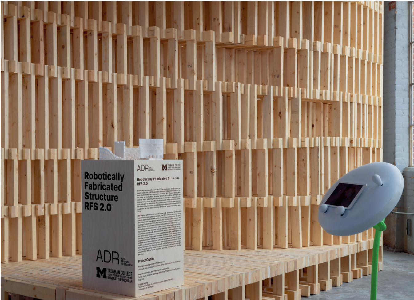
6 Fully assembled NLT structure, showing interior wall.
