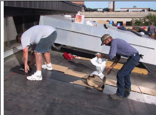
Modules glued on the rubber membrane of the roof
