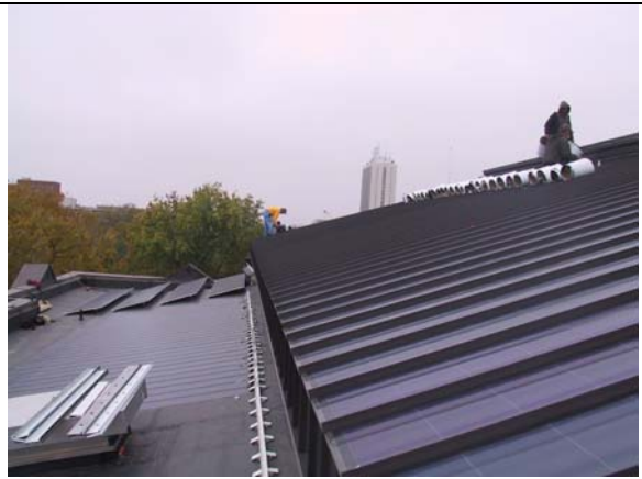
Modules installed on the metallic seam of the roof
