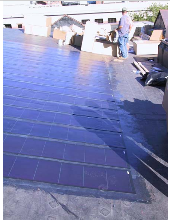
PVL Modules on Rubber Membrane
