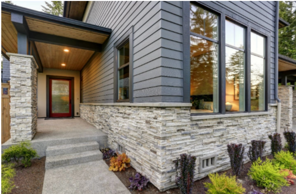
Figure 158: Habitat for Humanity's first 3D printed house owned by April Stringfield. Detail with house texture compared to stone veneer.
