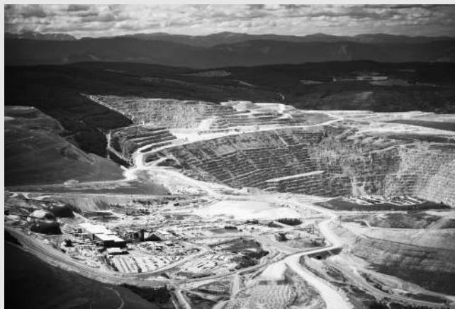
Figure Box 6.4.1 Highland Valley Copper Operation in British Columbia, showing the Lornex pit, beneficiation plant, and waste rock piles. Note the revegetated waste rock pile on the left behind the red domes. (Photograph courtesy of Teck Resources Ltd.) See color plate section.
