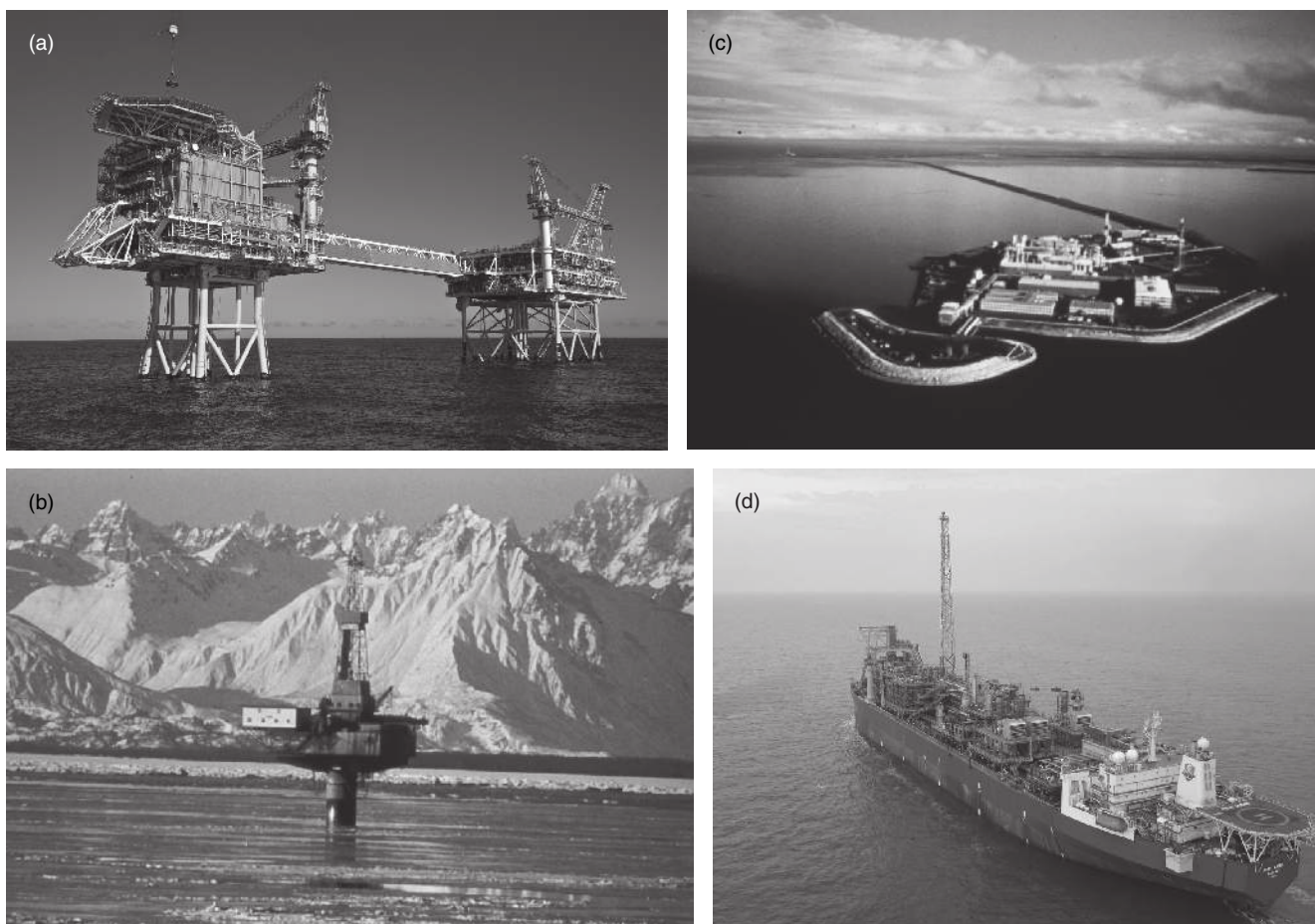
Figure 4.17 Offshore oil production in increasingly deep water. (a) The artificial ice-proof island that produces from the Endicott oil field near Prudhoe Bay on the north coast of Alaska was constructed in the mid 1980s for over $1 billion. The 445-acre (18-hectare) island has close spacing of wells designed to minimize its area and environmental impact. Initial oil production at a rate of about 100,000 bbl/day has declined to about 10,000 bbl/day today, and total production so far amounts to about 460 Mbbbl of oil (photo courtesy of BP America). (b) The Monopod platform, in 20 m of water in Cook Inlet, Alaska, began operation in 1967. Its single leg, which is less vulnerable to floating ice, has 32 wells that reach the entire oil field. With enhanced recovery methods that were applied in 2014, it produces about 2,900 bbl/day (photo courtesy of Chevron Corporation). (c) The Jasmine platform, at a depth of 81 m in the central North Sea, consists of a production unit with 24 slots for holes into the field and a living-quarters unit. The platform, with gross capacity of 140,000 bbl/day of oil equivalent (oil and gas), began production in 2013 (photo courtesy of ConocoPhillips). (d) In deep water where platforms do not work well, floating platform storage and offloading (FPSO) systems are used. The FPSO Aseng, shown here, began production from the Aseng field offshore Equatorial Guinea in November, 2011, at a water depth of about 1,000 m. The unit produces 80,000 bbl/day using injection of 150,000 bbl of water and has a storage capacity of 1.695 Mbbbl (photo courtesy of Glencore Ltd.). See color plate section.
