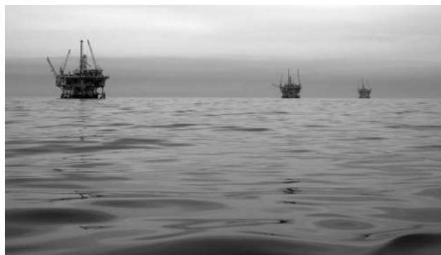
Figure 5.5 Oil fields in the Santa Barbara Channel, just offshore from the city of Santa Barbara, California, are an important source of US oil production. The Dos Cuadras field, which is served by Platforms A, B, and C shown here, is in federal offshore land, just beyond the state limit. The field is at a depth of 2,000 to 3,500 feet and has produced more than 260 Mbbl of oil since it was discovered in 1968. The field is outside the 3-mile limit and therefore is administered by the US federal government. A spill of almost 100,000 barrels from this field in 1969 was a catalyst in the US environmental movement. Although this was a large spill, it is much smaller than the natural oil seepage that has been going on in the Channel for the last few hundred thousand years (photograph courtesy of Doc Searls).
