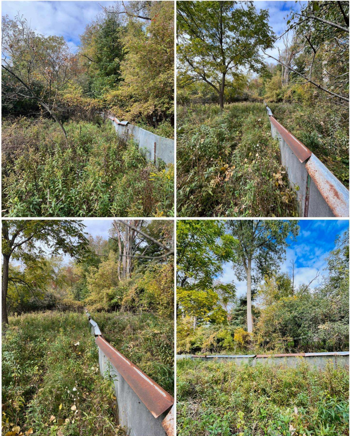
Figure 22: Fence found on the northern edge of Site 2, during the study.
