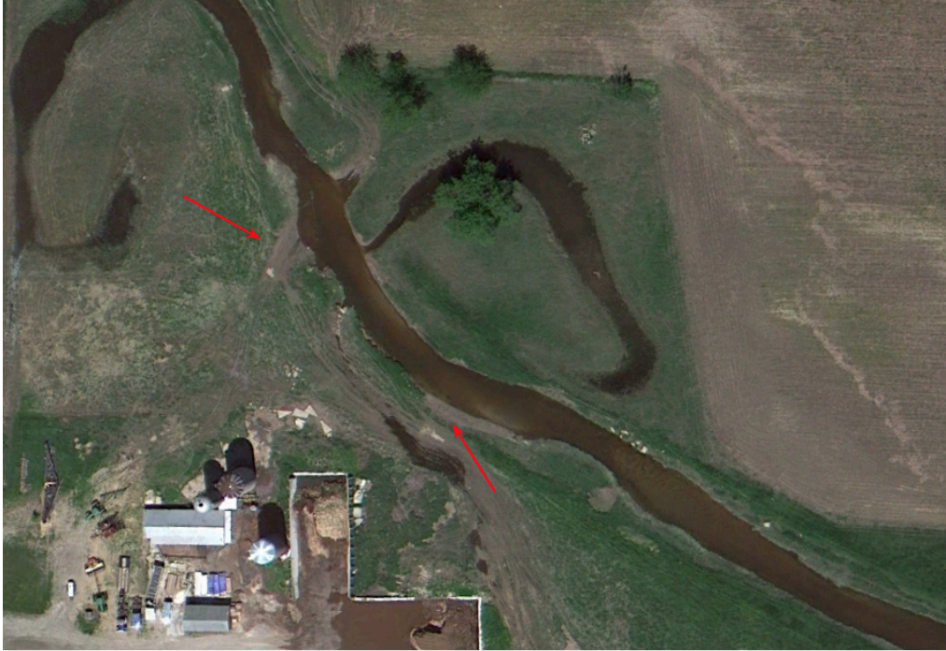
Figure 11: Arrows indicate areas of bare soil where animals may have access to the stream. Banks appear disturbed.
