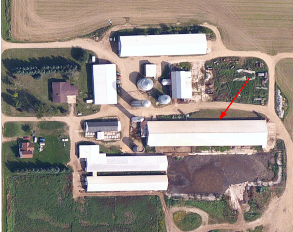
Figure 3. Larger operation with typical white structures of an AFO.
