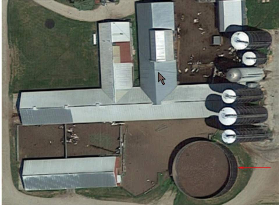
Figure 14: Arrow indicates above ground manure storage structure.
