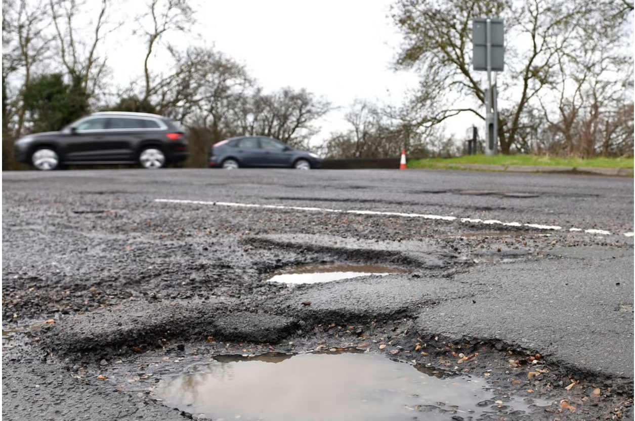
Figure 1.1: Potholes Formation.[16]
