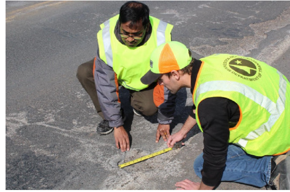
(b) Potholes Inspection Manually [38]
