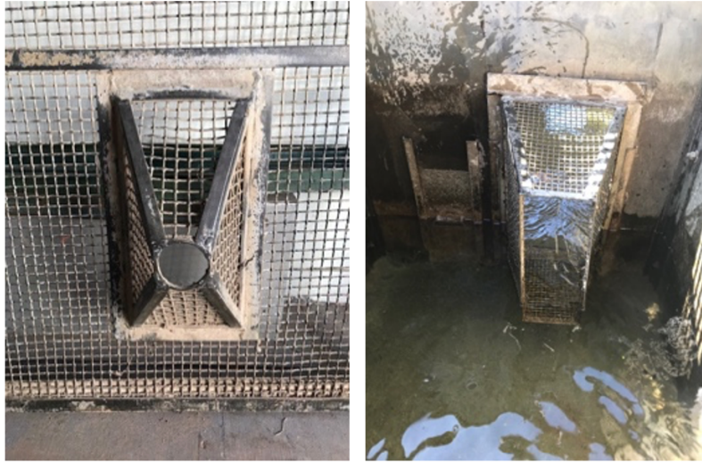
Figure 5.1: Mesh face trap (left) and solid face trap (right) examples. View from inside trap facing downstream.
