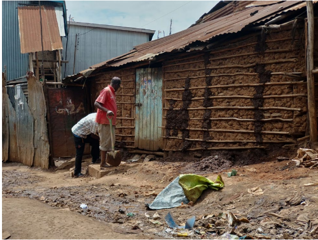
Figure 5.4: Residents working on church/meeting hall building. Image by author.
