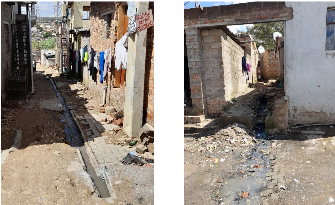
Figure 4.8: Examples of drainage systems constructed by residents using local knowledge and labor. Images by author.
