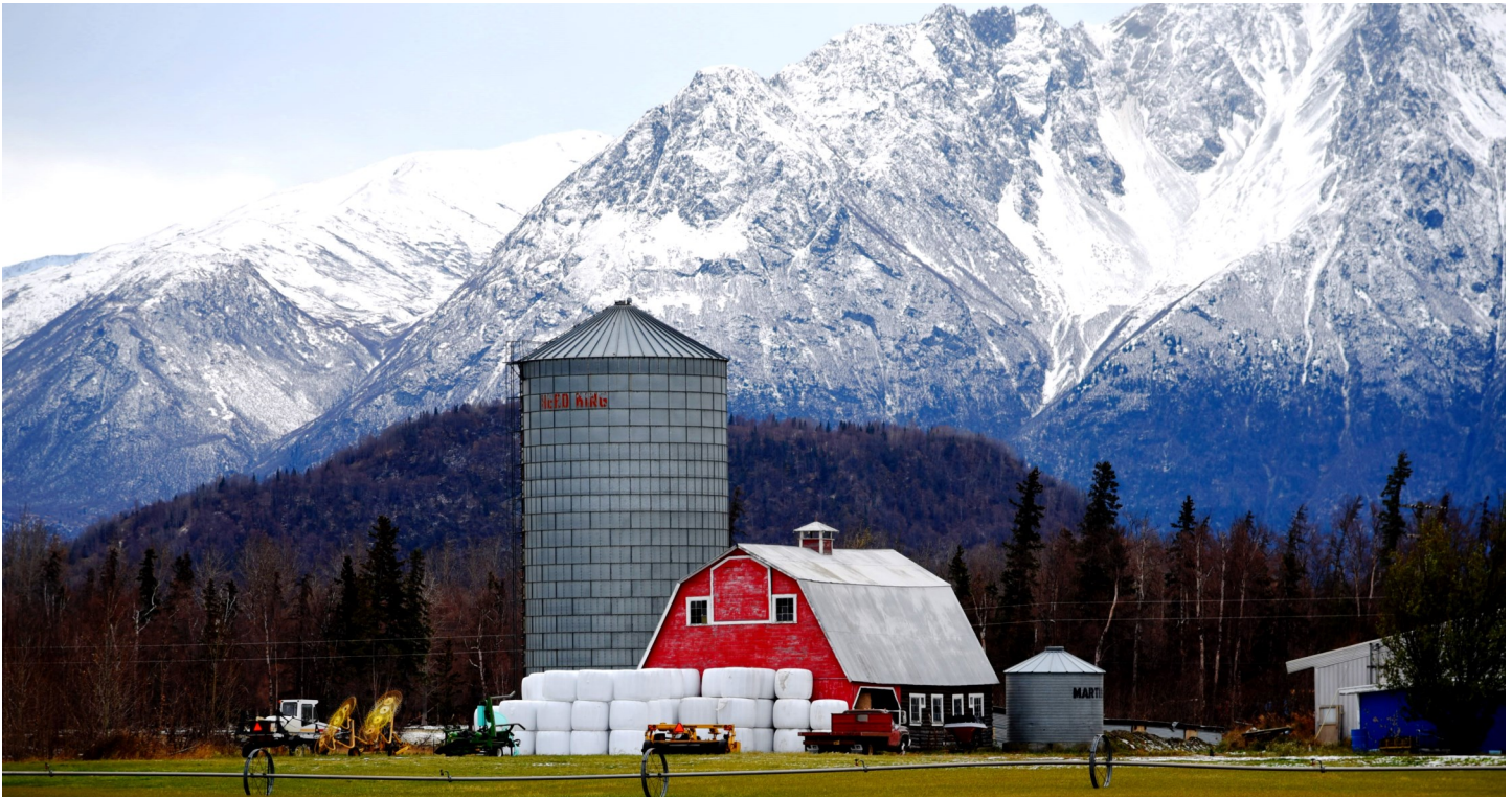
Figure 9. Konig, J. (2021). Farm Structure in Palmer, Alaska. Flickr.
