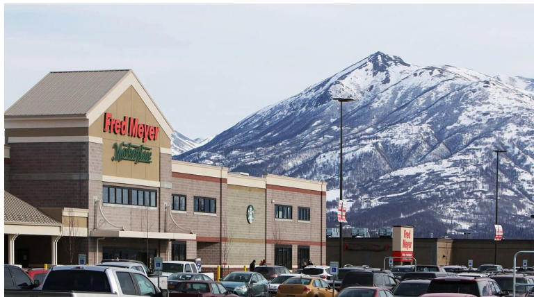
Figure 23. Fred Meyer. (n.d.). Barghausen Consulting Engineers,
