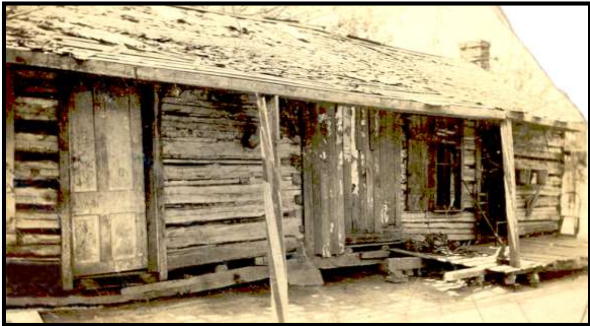
Farm worker residential quarters.
