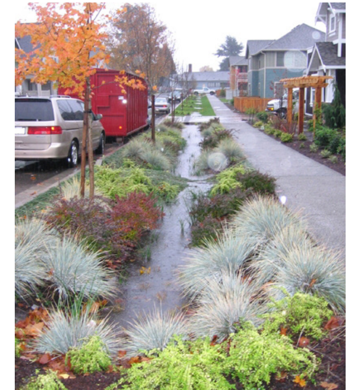
Figure 2.11 Roadside rain garden
