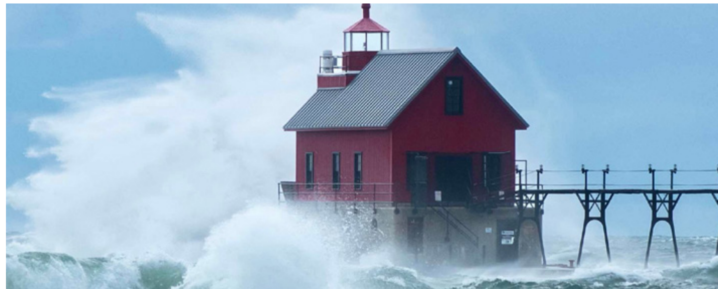
Figure 2.1 South Haven, MI Large Waves, High Winds, and Beach Erosion
