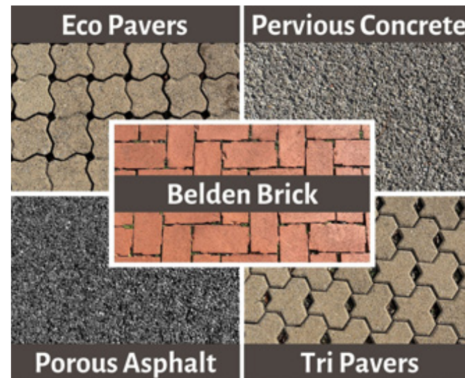
Figure 2.12 Different types of pervious pavement
