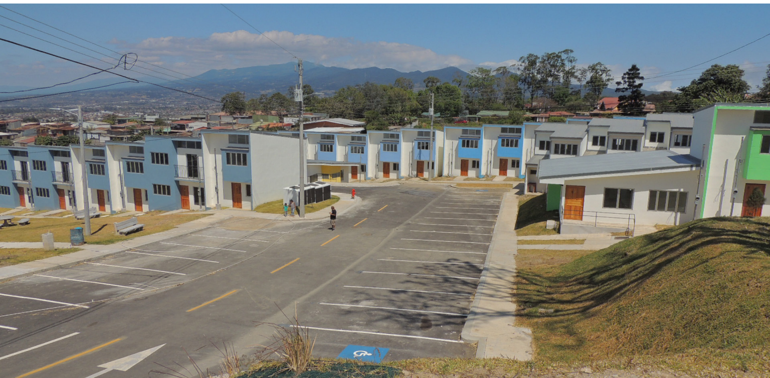
Figure 05.16 FUPROVI self-managed housing project “Linda Vista” in the Goicoechea region of San José
