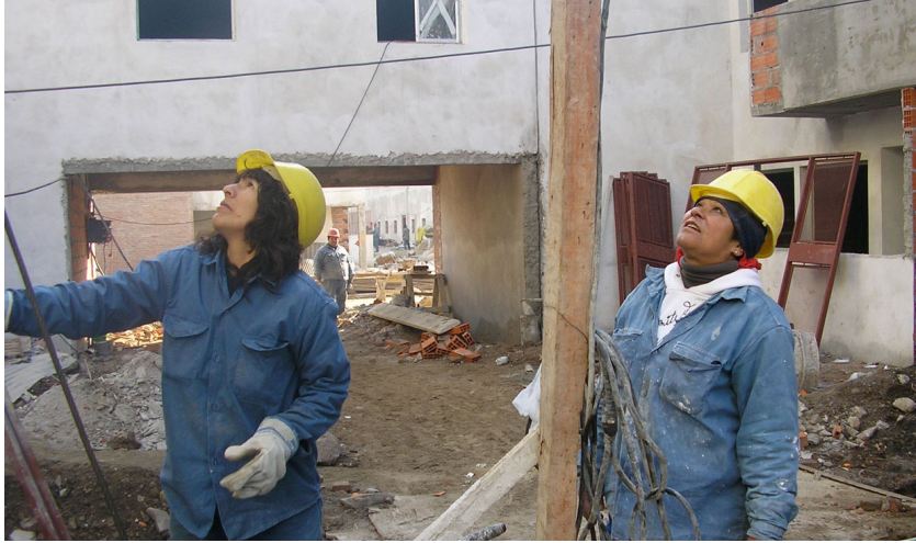
Figure 05.12 Member-Workers from Movimiento Territorial de Liberación Construct their Future Homes.
