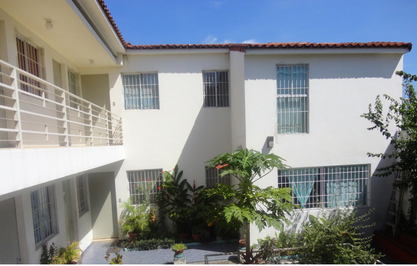
Figure 05.18 ACOVICHSS cooperative housing project in San Esteban
