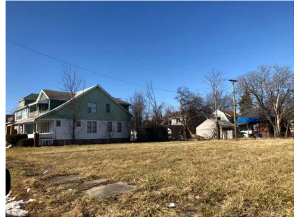
Figure 3.8: DLBA-owned structure with a vacant sidelot in Northeast
