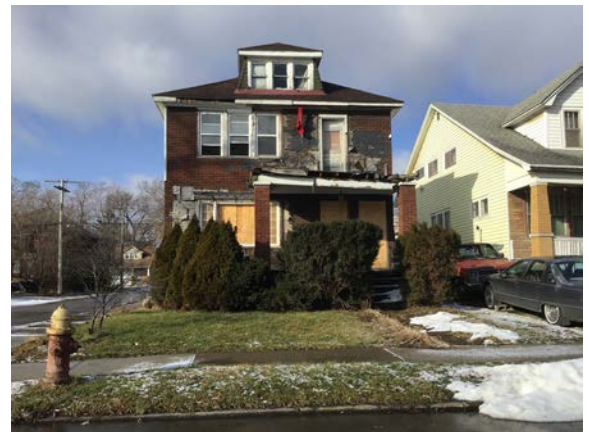
Figure 3.1: DLBA structures in Claytown
