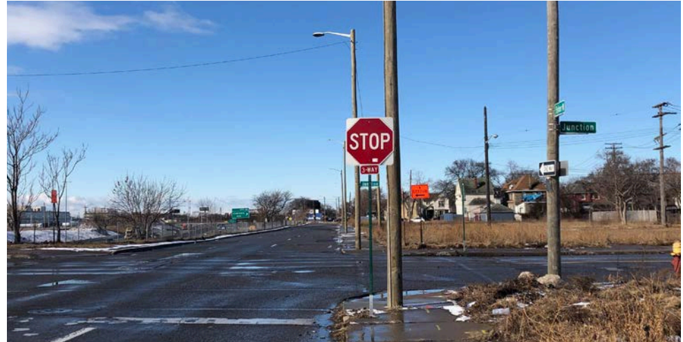
Fisher Service Drive that runs parallel to I-75.
