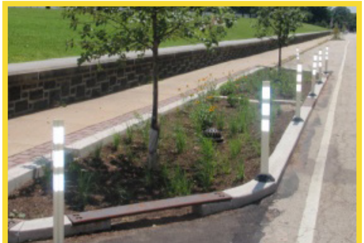
Figure 3.11: A stormwater bumpout in the public right-of-way Source: Philadelphia Water Department
