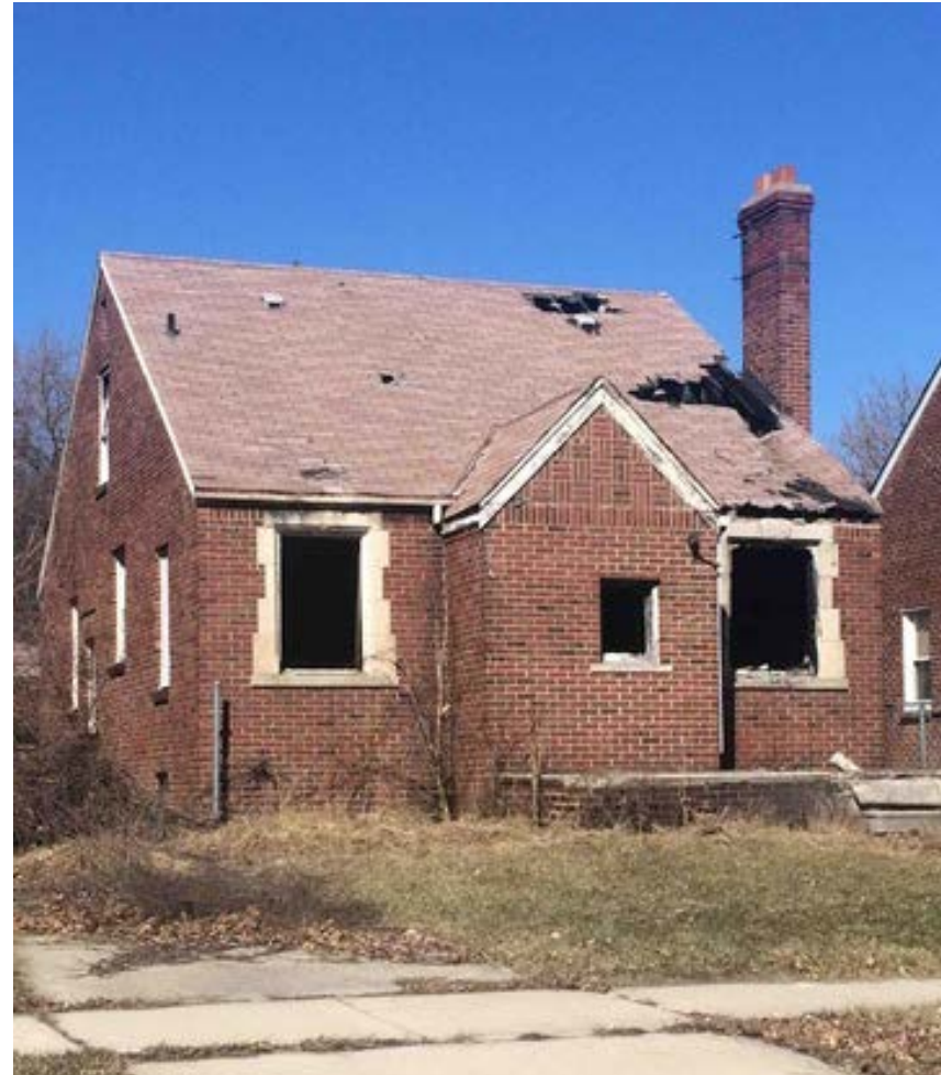
Figure 3.13: Some structures suggested for demolition are not in the demolition pipeline.
