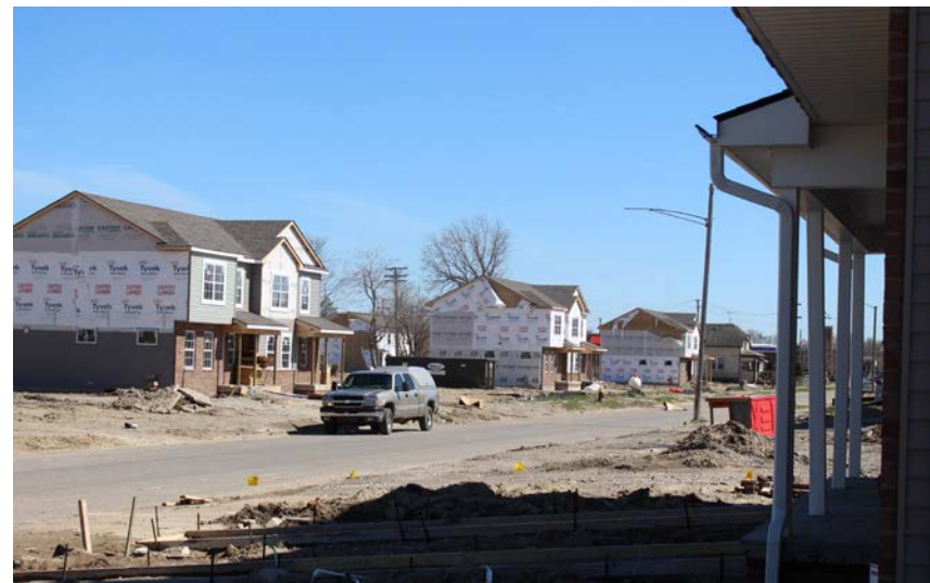
Figure 2.9: Mack-Ashland supportive housing was under construction in April 2017.
