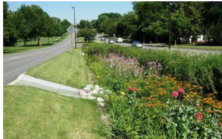
Figure 3.28: Chandler Park Drive's median could be improved with a GSI installation.
