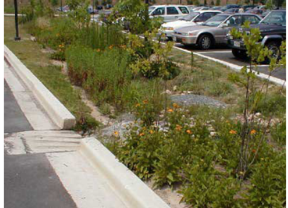
An example of Low Impact Design, which incorporates bioretention swales into otherwise impervious parking lots. Source: http://www.water-research.net/images/bioretentionparking.jpg
