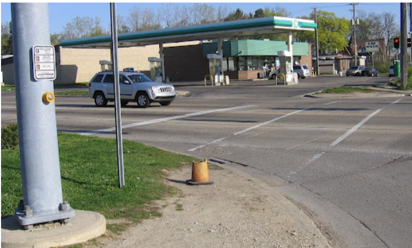
Figure 1.19: Intersection of Washtenaw and Goldside, Lacking Sidewalks and Curb Ramps
