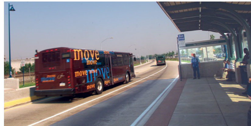
Figure 3.15: Pittsburgh's East Busway
