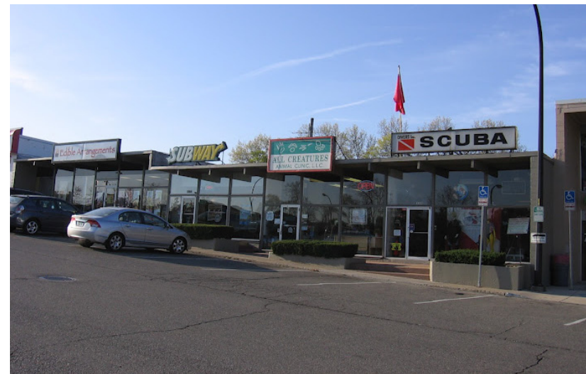
Figure 1.10: Small Strip Commercial Development, Ann Arbor.
