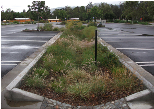
FIGURE IV-22. LANDSCAPING ISLAND IN A GREEN PARKING LOT | SOURCE: GONZALEZ, C. (2011). L.A. ZOO'S NEW WATERSHED-FRIENDLY PARKING LOT. RETRIEVED APRIL 21, 2016, FROM HTTPS://LACREEKFREAK.WORDPRESS.COM/2011/05/21/LA-ZOO'S-NEW-WATERSHED-FRIENDLY-PARKING-LOT/
