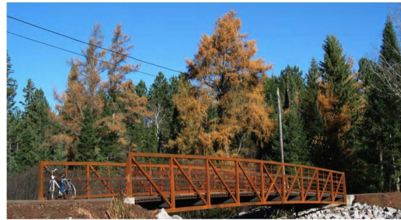
FIGURE IV-24. MULTI-MODAL BRIDGE IN CONOVER, WISCONSIN | SOURCE: CURRIE, J. (2015). MOVING TOWARD A BIKE-FRIENDLY EASTERN VILAS COUNTY. RETRIEVED APRIL 21, 2016, FROM HTTP://WISCONSINBIKEFED.ORG/2015/12/16/NEW-TRAILS-IN-EXPANDING-IN-EASTERN-VILAS-COUNTY/
