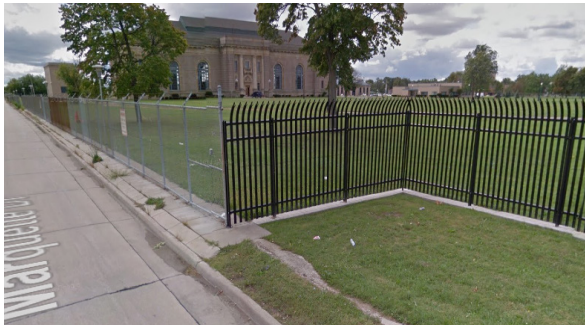
FIGURE IV-14. FENCE ALONG WATERWORKS PARK | SOURCE: MARQUETTE DRIVE. (N.D.). GOOGLE STREETVIEW.
