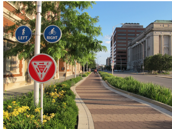
FIGURE IV-20. BIOSWALES ALONG A BIKE LANE | SOURCE: BIKE OKC. (2014). BIOSWALES ALONG CYCLE TRACKS ON THE INDIANAPOLIS CULTURAL TRAIL. RETRIEVED FROM HTTPS://BIKEOKC.WORDPRESS.COM/2014/01/
