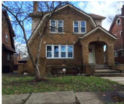
Figure 7.2 3485 Courville Street (right)
