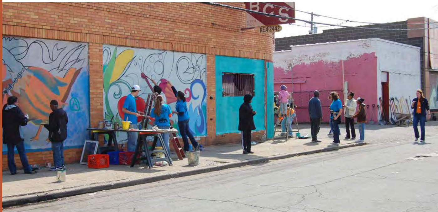
Figure 4-3: Community residents and University of Michigan students partner to improve building facades in Detroit. Source: University of Michigan, Edward Ginsberg Center.
