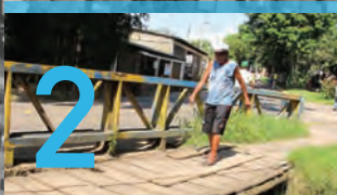
2 BRIDGE AT ENTRANCE
