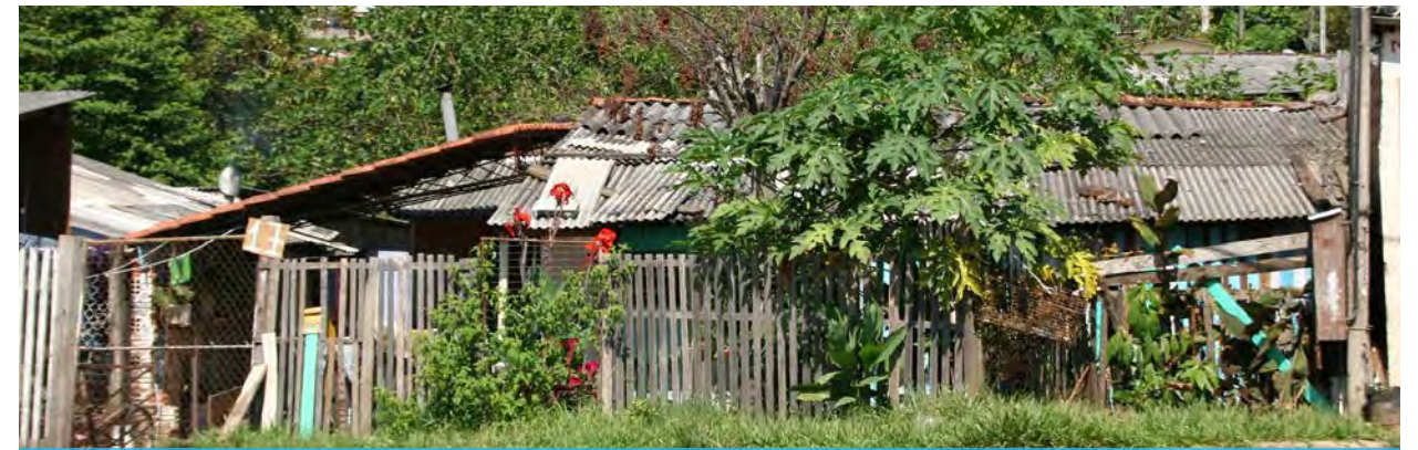
Many residents use a variety of materials, such as unfinished wood and metal sheeting (as illustrated above) to construct homes that are not as resilient to flooding and weather as those built with more traditional material.
