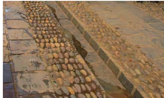
Example of stone pavers and a small open channel to guide stormwater on a sidewalk in Cusco, Peru.
