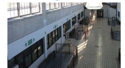
Nottingham Water Treatment Plant, Collinwood Neighborhood
