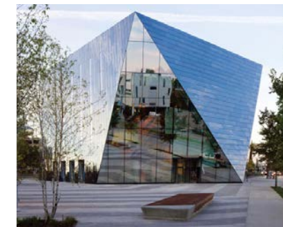
Ground Source Heat Pumps (geothermal wells) are used to heat and cool the museum by geothermal wells located under the adjacent plaza. Image: MOCA Cleveland Source: Sustainable Cleveland 2019
