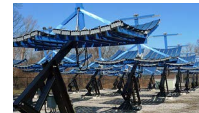
Parabolic mirrors can focus sunlight and produce electricity and thermal energy to heat the greenhouse. Image: Solar Photovoltaic Concentrator System at the Rockefeller Park Greenhouse in Cleveland, Ohio.
