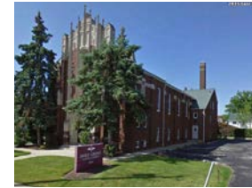
Holy Grove Baptist Church Completed.
