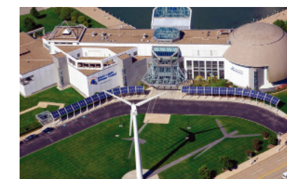
Onshore wind turbine w/ peak output of 225KW at wind speeds of 31 mph. Solar array canopy producing an annual average of 100KWh/day at the Great Lakes Science Center, Cleveland. Image: Great Lakes Science Center, Cleveland Source: Sustainable Cleveland 2019
