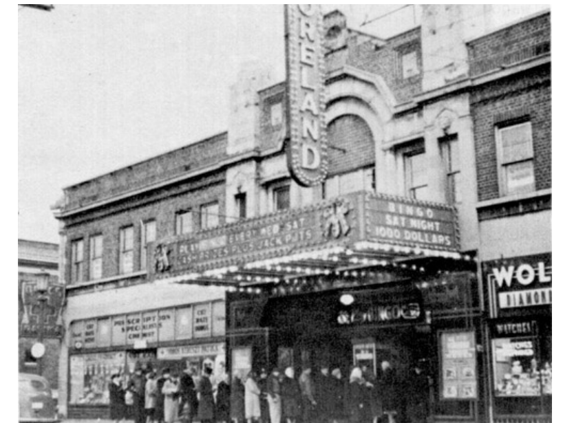
Original facade and use of The Moreland Theater in the 1920's.
