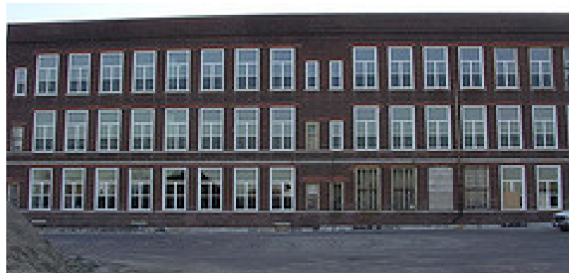
Harvey Rice Elementary School before rehabilitation
