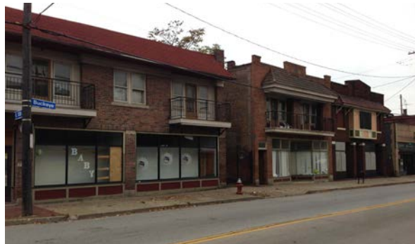
B. E. 120th and Buckeye Rd. (South)
