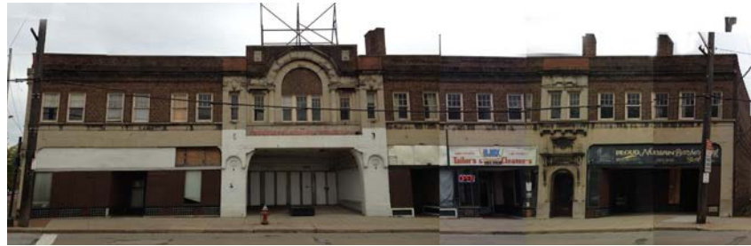
Existing Moreland Theater Condition
