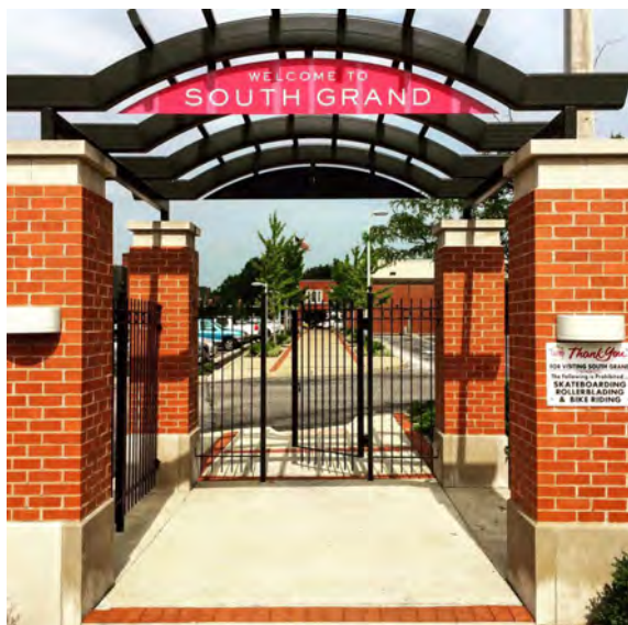
The South Grand CID redeveloped a parking area for residents and visitors. Photo: South Grand Facebook page
