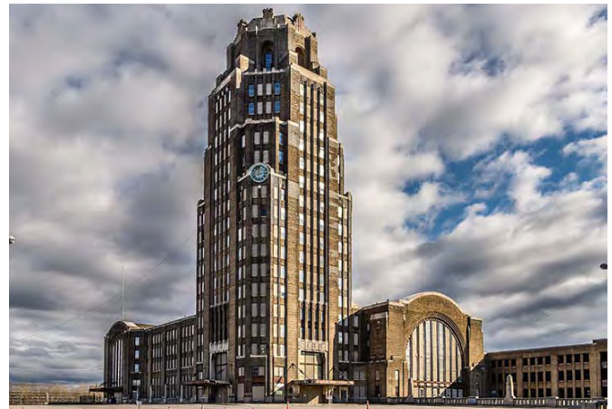
The Buffalo Central Terminal lies at the heart of Broadway-Fillmore. The city and state are currently planning the redevelopment of the landmark. Photo: Buffalo Central Terminal website
