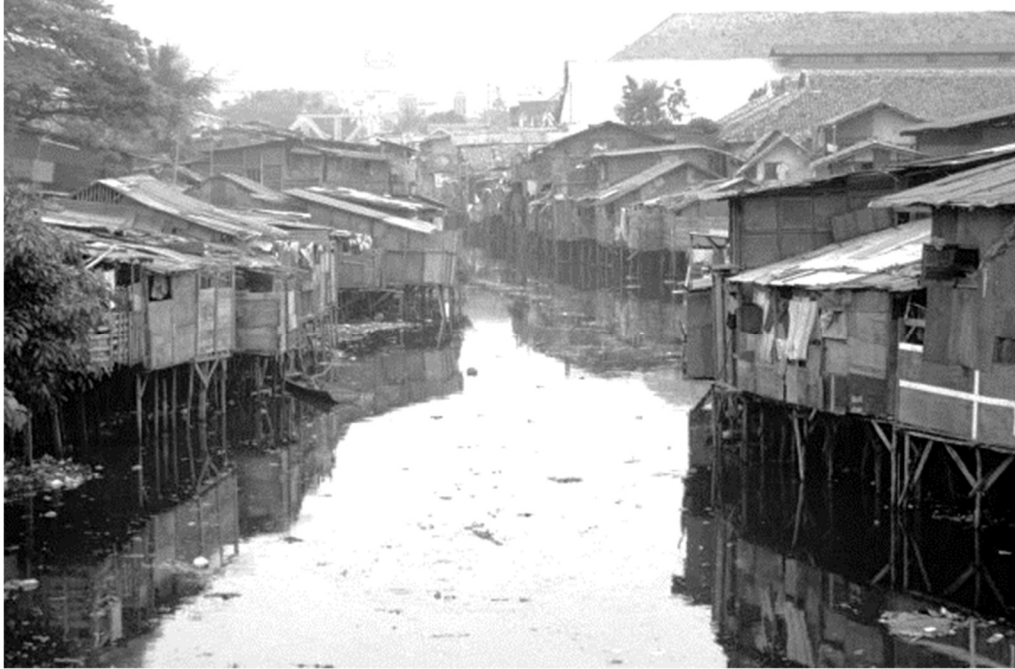
Figure 9. Illustration of the pre redevelopment condition of the riparian slums in Jakarta. Image source: https://konservasidasciliwung.wordpress.com/sempadan-ciliwung/berita/ .
