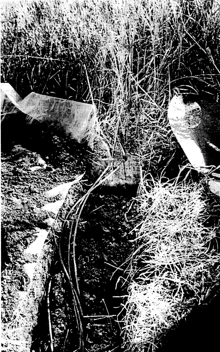
Figure 5.9: Insertion of the soil temperature probes. At the time of this picture, I had already inserted the probes in the side of the trench and refilled it, burying the 64, 32, and 16 cm probe cables. Cables leading to the 2, 4, and 8 cm deep probes protrude from the side of the trench.
