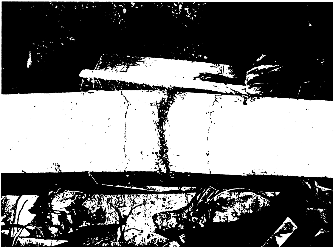
Fig. 3.3 (i)- Specimen B9 at failure.
