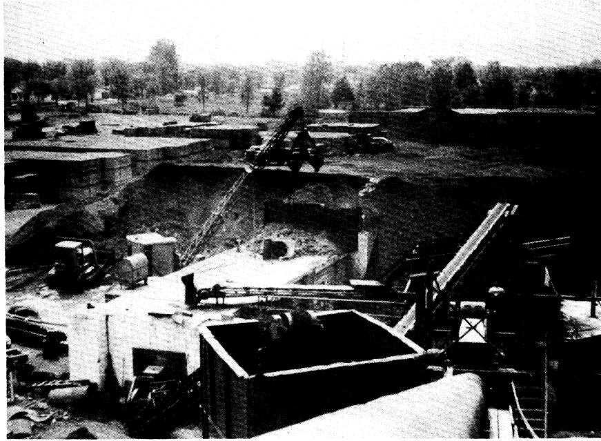
Figure 1. Cinder Aggregate Processing Equipment.
