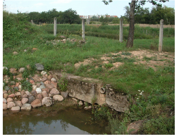
Figure 60. Overflow pipe from pond.
