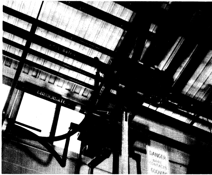
(a) Overhead Knife Switches
