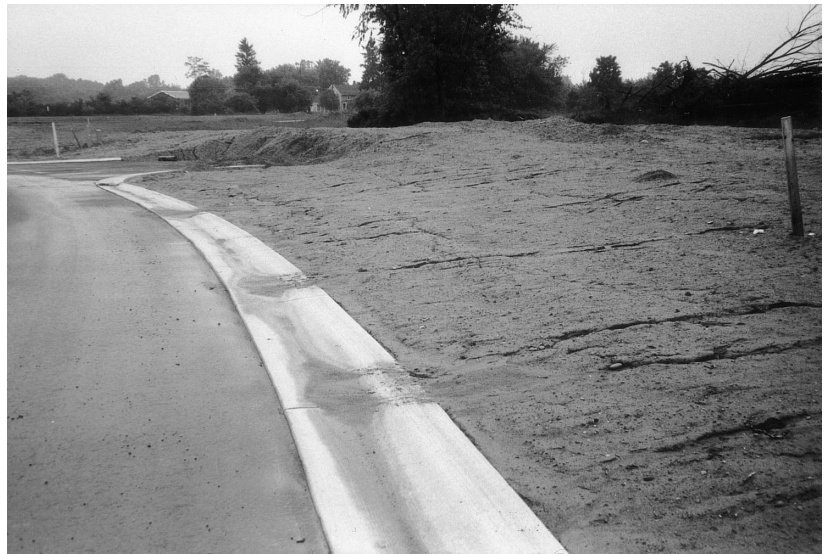
Figure 4. Inadequate slope stabilization.
