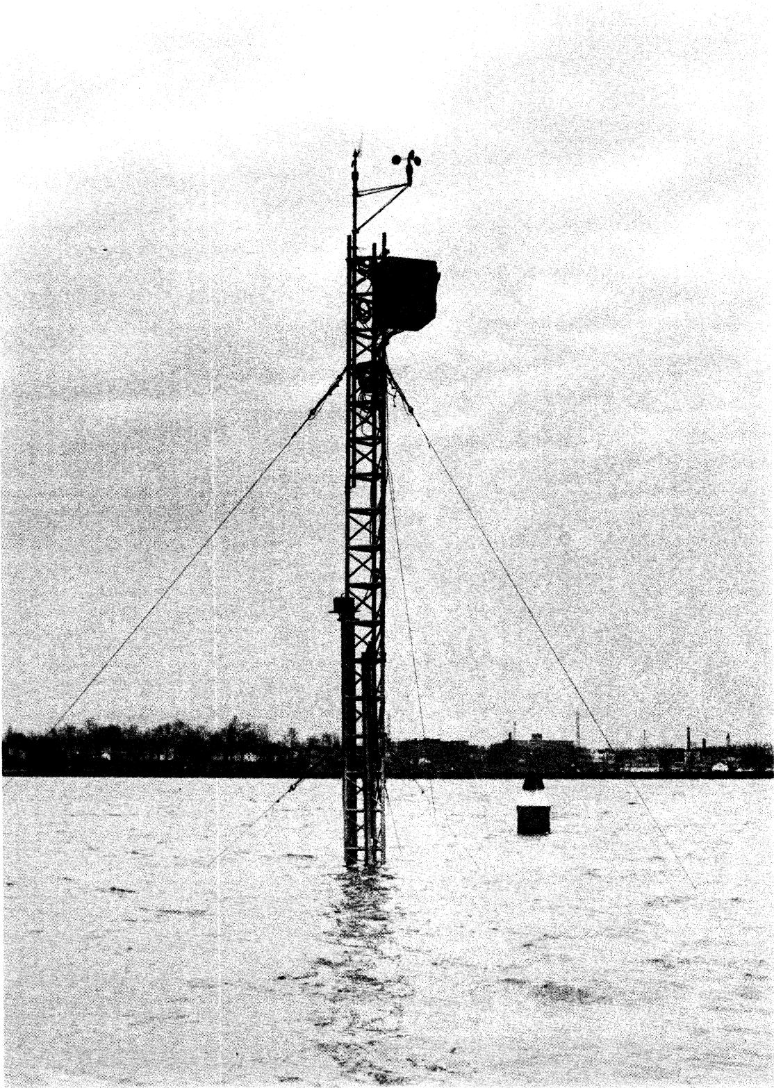
Figure 9. The 50 ft. guyed tower mounted on the bottom of Lake Erie. The thick dark line in the background is the East Breakwater Shorearm.
