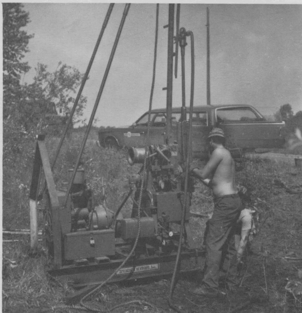
TEXT-FIG. 59 -- Drilling through the Norwood Shale west of Beebe School. Here the core barrel is being hoisted from the hole by McDonald and Cregger.
