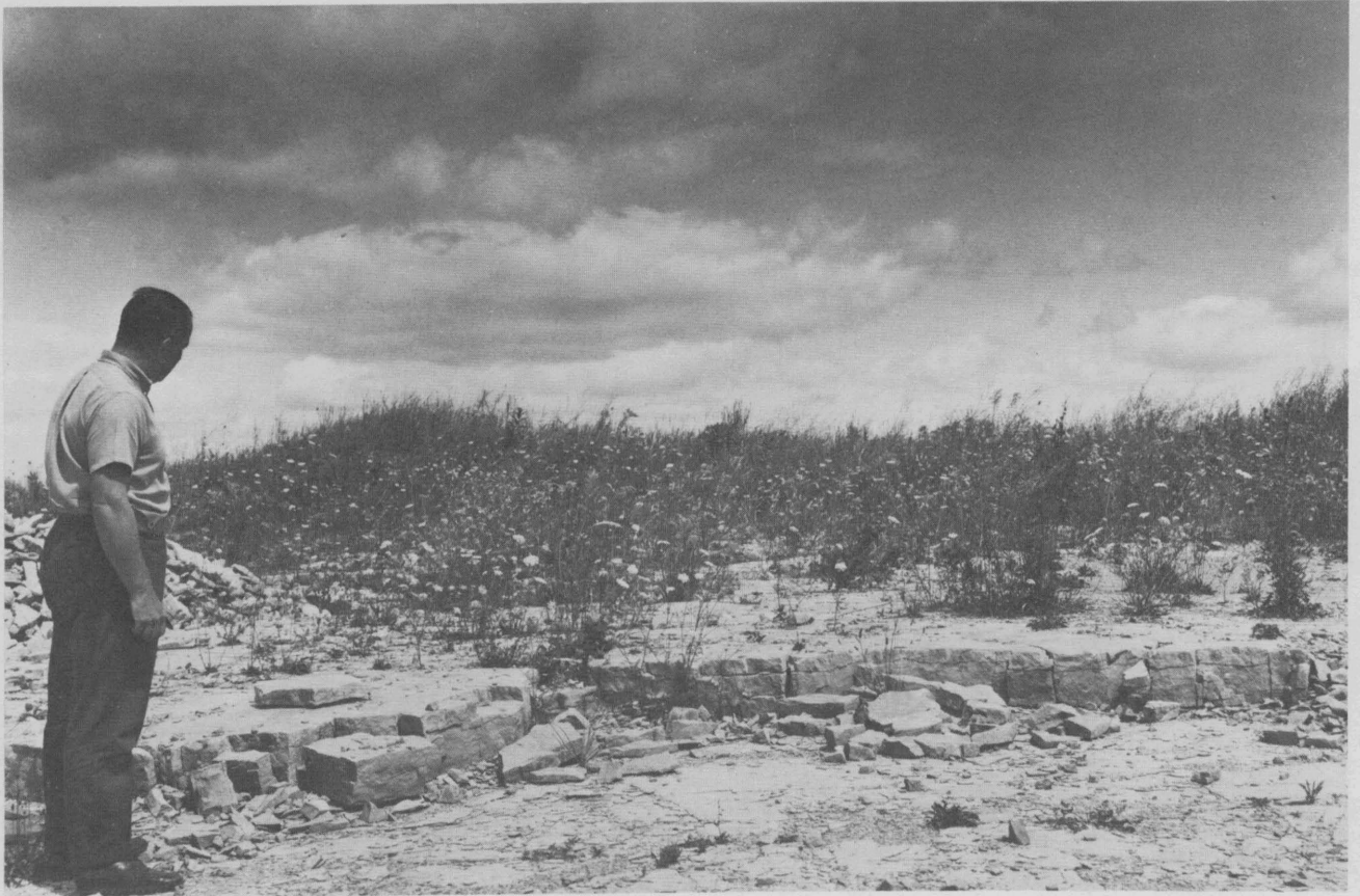
TEXT-FIG. 27 -- Koehler Limestone exposed in Onaway Stone Company Quarry. Locality 34-2E-5 N. The jointing of the limestone here is used to advantage in selective quarrying for building stone. Karl Kutasi, now retired, looks on a temporarily abandoned border of the quarry area. Photograph by Kesling, 1969.
