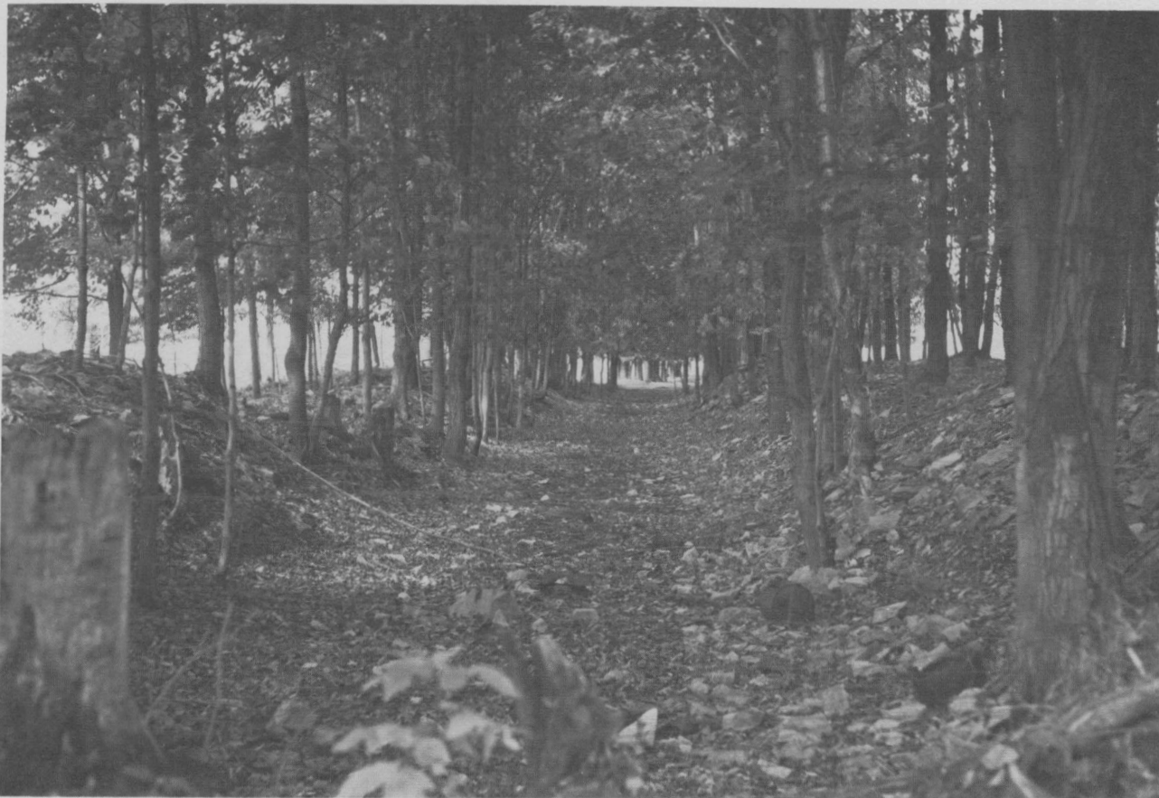
TEXT-FIG. 36 --- Gravel Point Formation exposed in a long-abandoned railroad cut east of the site of Gorbuts School and southwest of Le Grand Quarry. Locality 35-1W-33 N. The limestone here is considered to be above the Gorbuts Member. Photographed by Kesling, 2 Oct 1975.
