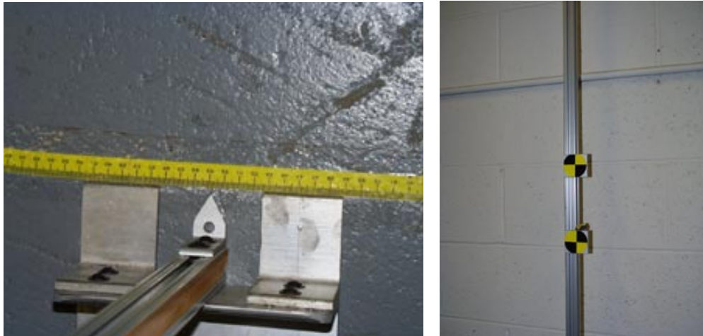
Figure 2. Measurement tape and sighting pole.
