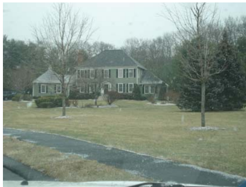
Figure 4.10: Olde North Mill, Hopkinton, MA
