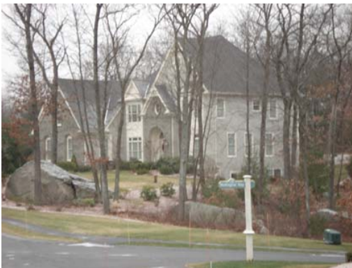
Figure 4.9: Olde North Mill, Hopkinton, MA
