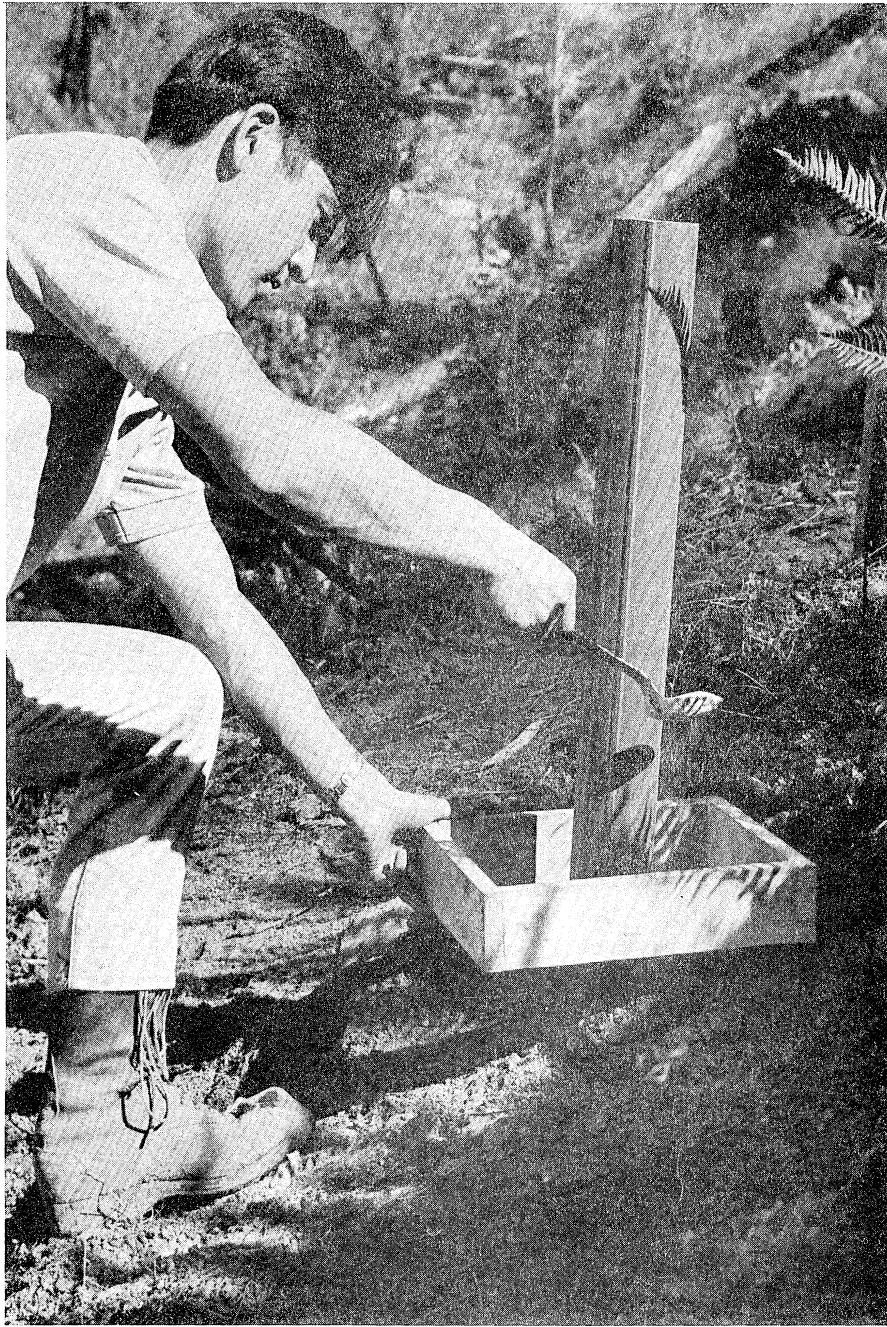
Figure 20. Backfilling around slope indicator casing using 'single grain, air dropping' technique.
