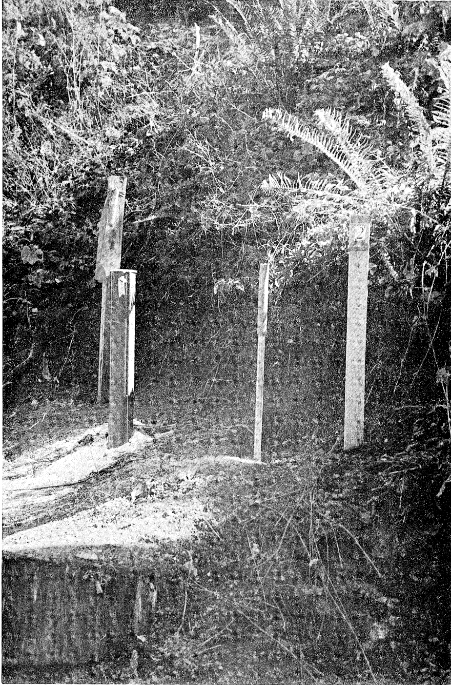
Figure 22. View of a typical inclinometer tube installation.
