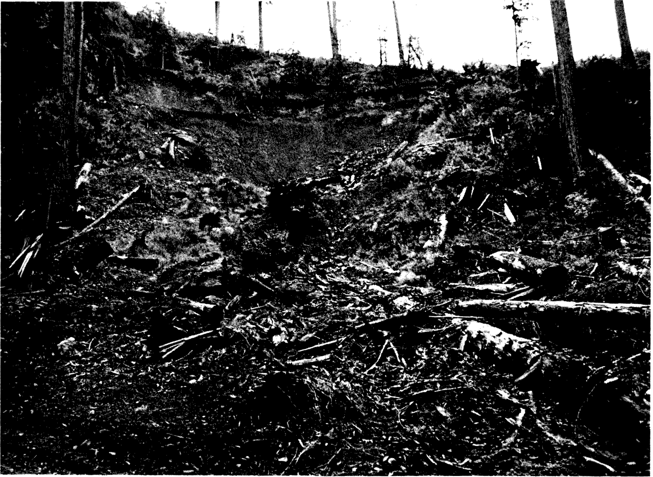
Figure 18. Slide occurring in a disturbed area, H. J. Andrews Experimental Forest.
